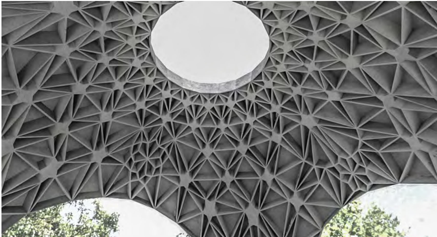
Structural muqarnas of hasht behesht palace
